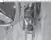
Connect Blue Wire to Safety Switch on Drier
