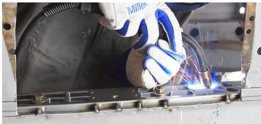
Figure 17 - Finish Weld Adapter Plates & Floating Stanchions
